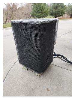
There are steps you can take to protect your facility from hail. Hail damage to roof coverings and roof mounted equipment such as air conditioners, vents and skylights is common. Protective shields commonly referred to as "hail guards" or "hail screens" can be installed to protect this fragile equipment, both ground and roof mounted, from hail stones.
